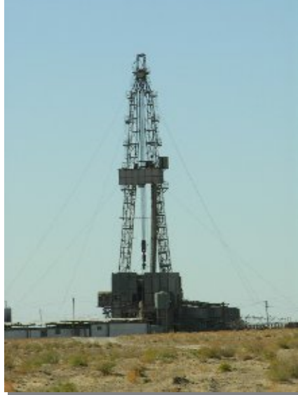
View of oil drilling rig near Muynak
